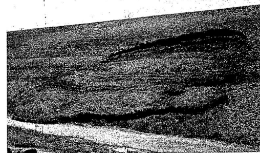
FIGURE 4.32 This small, tongue-shaped earthflow occurred on a newly formed slope along a recently constructed highway. It formed in clay-rich material following a period of heavy rain. Notice the small slump at the head of the earthflow. (Photo by E. J. Tarbuck)
