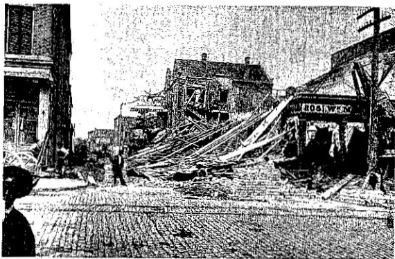
FIGURE 8.A Damage to Charleston, South Carolina, caused by the August 31, 1886, earthquake. Damage ranged from toppled chimneys and broken plaster to total collapse. (Photo courtesy of U.S. Geological Survey)
