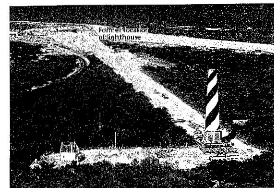
FIGURE 15.29 When the lighthouse at Cape Hatteras, North Carolina, was built in 1870, it was situated 457 meters (1,500 feet) from the shoreline. By 1970, waves began to lap just 37 meters (120 feet) from its base. In order to save the historic structure, it was moved 488 meters (1,600 feet) back from the shore. At the current rate of shoreline retreat, the lighthouse should be safe for another 50 years. (Photo by Reuters/Stringer/Getty Images, Inc.—Hulton Archive Photos)
